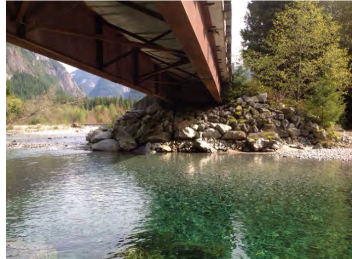
Left Bank Abutment when facing downstream
