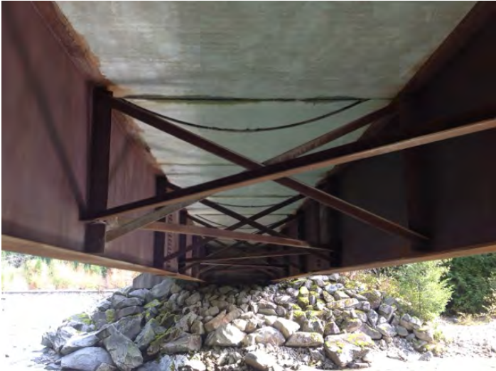
deck seals all pushed through
