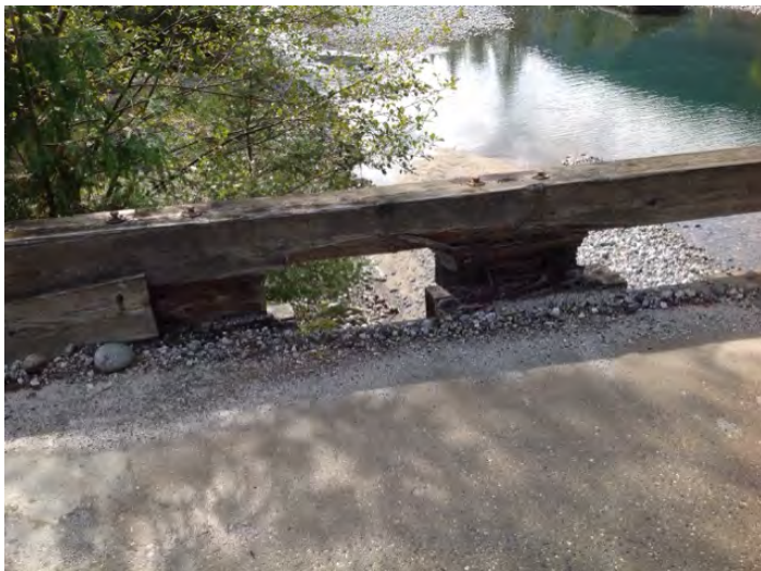
guardrail damage
