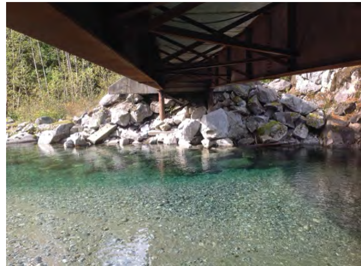
Right Bank Abutment when facing downstream
