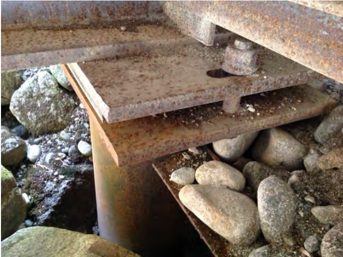
bearing bolts at full extent of slot
